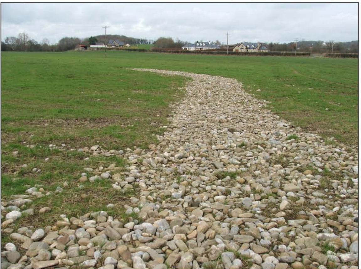
Plate 12 Field 9 facing north, showing gravel laid over pipe trench
