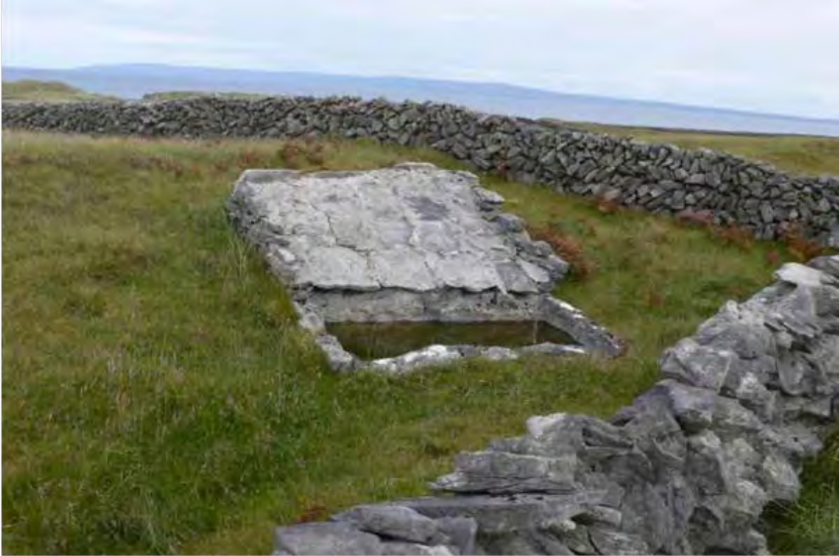
Limestone-built water collector and field walls, Inis Meáin, Co. Galway (Barry O'Reilly)
