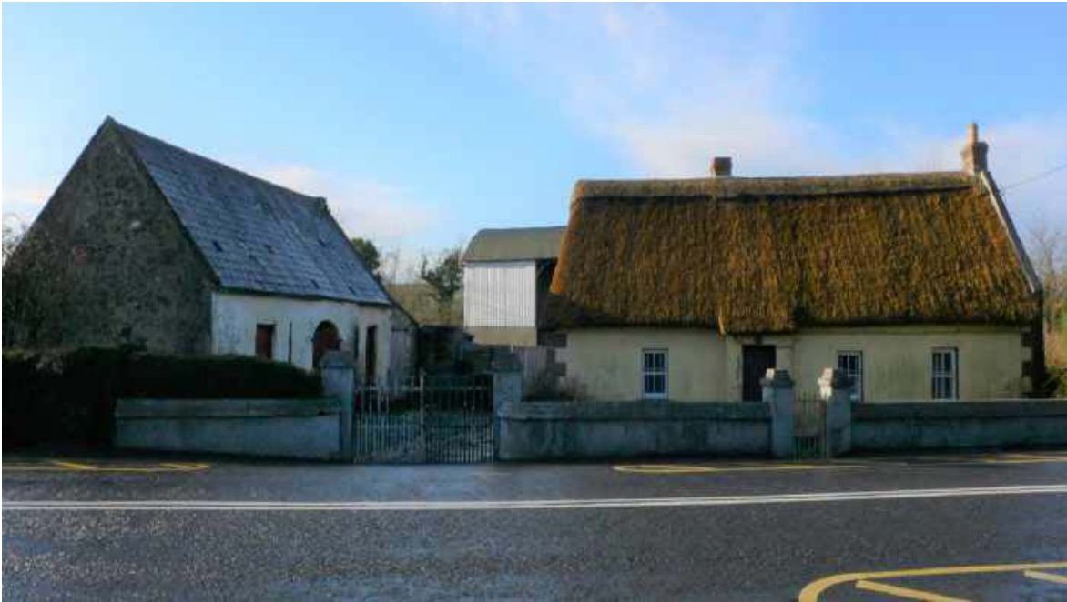
Farmyard at Oola, Co. Limerick, displaying a range of vernacular buildings, features and materials (Barry O'Reilly)
