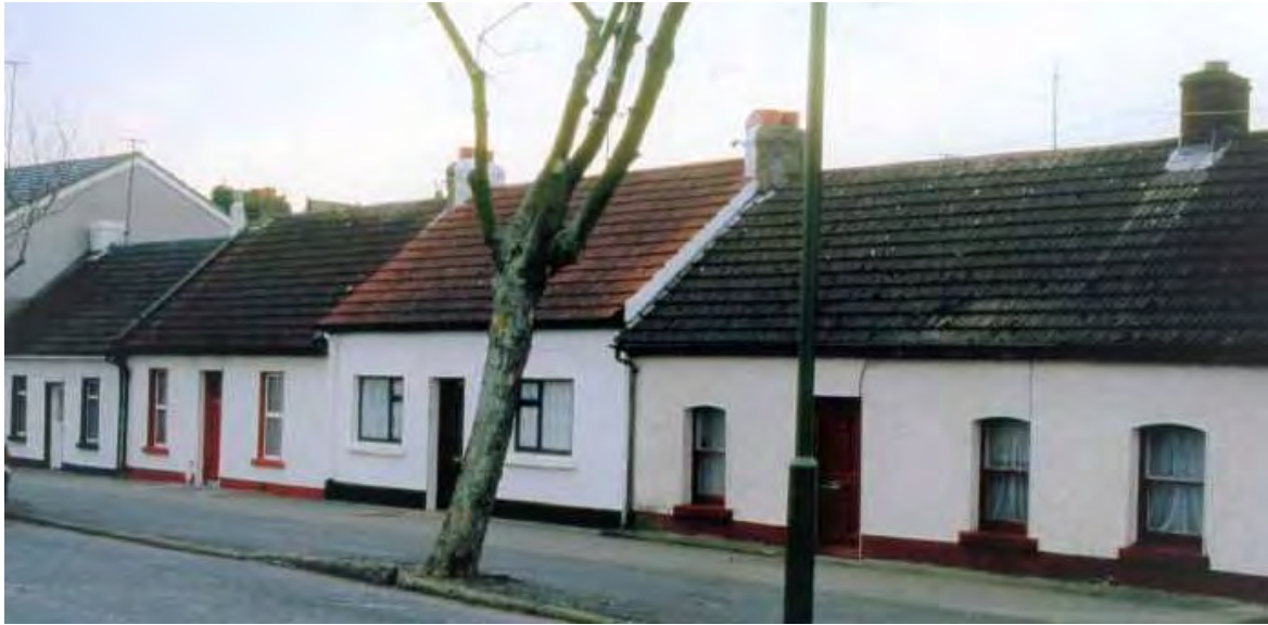
Urban vernacular housing, Strand Street, Skerries, Co. Dublin (Barry O'Reilly)
