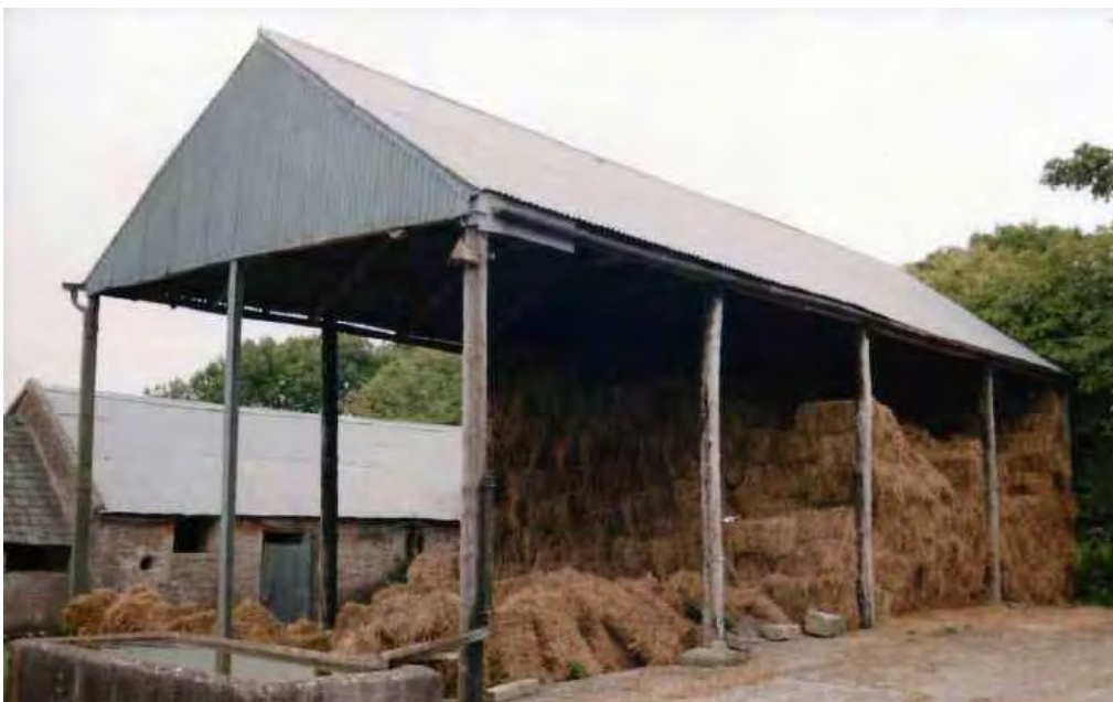
Hay barn of informal construction, near Barringtonsbridge, Co. Limerick (Barry O'Reilly)
