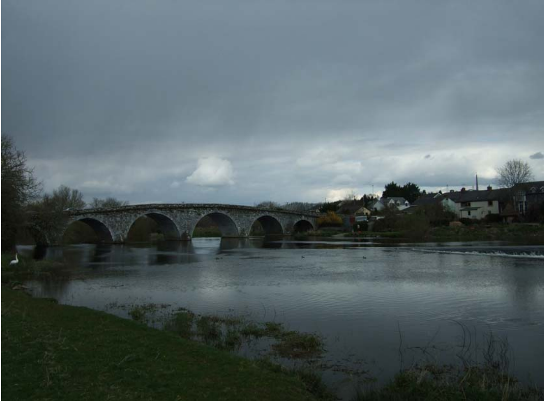
Figure 4: Looking northeast across river towards the bridge
