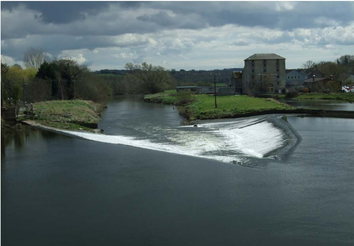
Figure 3: Mosse mill with weir to foreground
