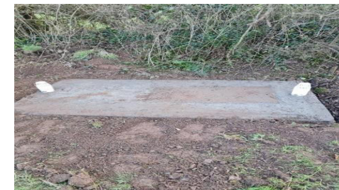
New Cover provided to existing Septic Tank following inspection
