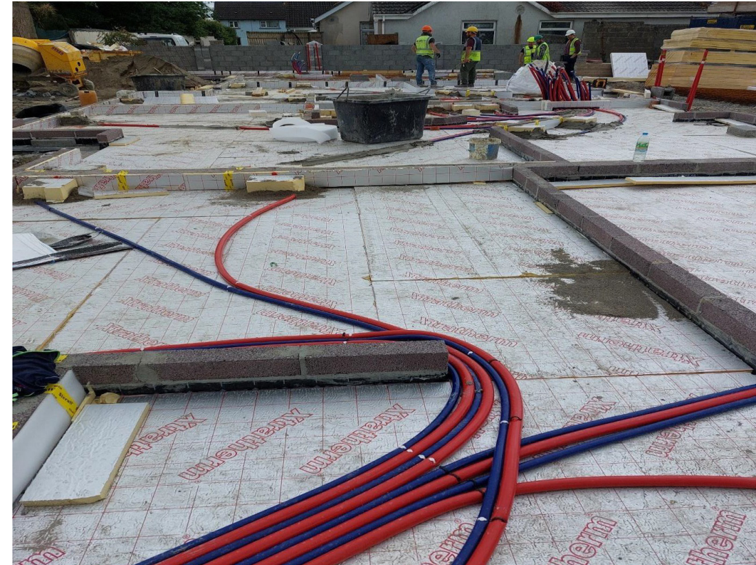
6 units at Golf Links Road – infill scheme, substructure complete
