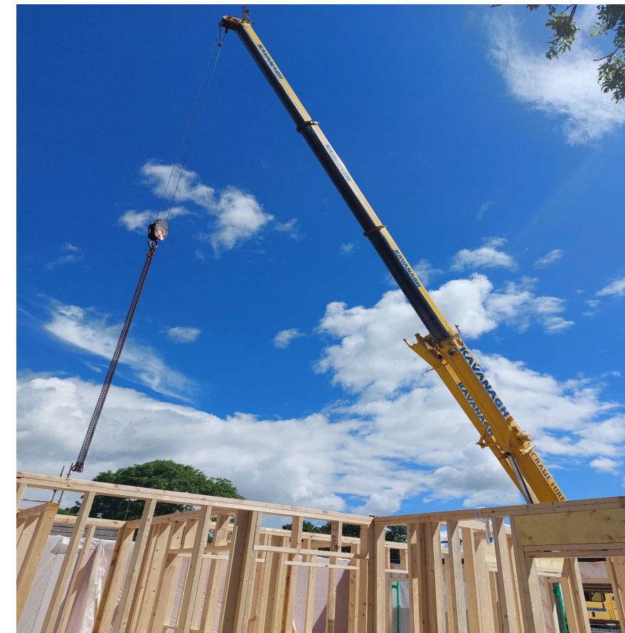
Erection of timber frame at Inchacarron Mullinavat. Low Carbon Construction
